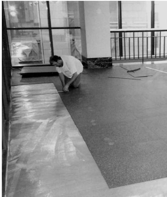
Square Cut Glue Down Installation
